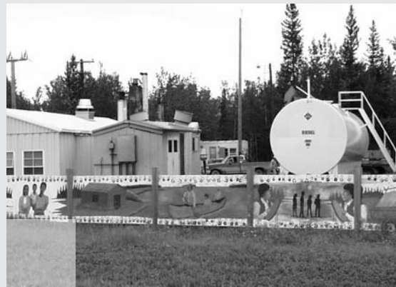
Fort Providence diesel plant.
