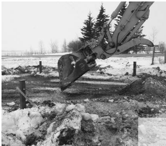
Radway substation remediation.
