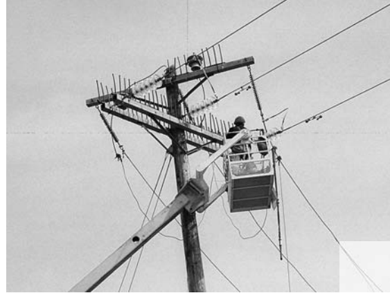
Bird guards being installed on a corner structure.
