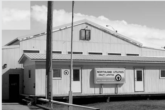
The Hay River diesel plant.
